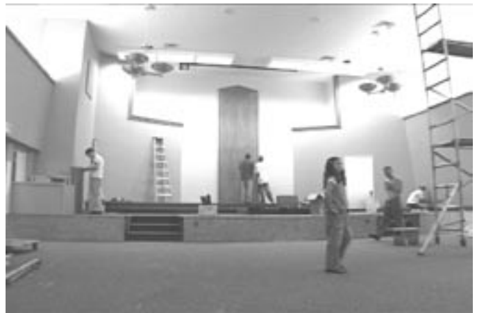
Church members help dismantle the fifth-floor chapel.
